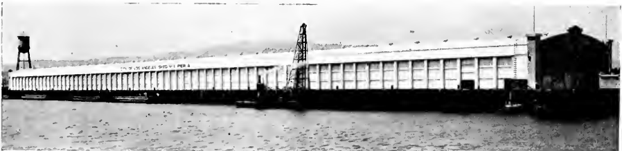
Shed No. L, Pier A, at which the American-Hawaiian S.S. Co. berths. The shed is 1005 feet long and 100 feet wide, and was the first wharf and shed built by the City of Los Angeles.
